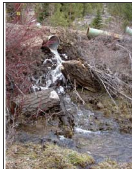
PHOTO #2: Fish Blockage of Alder Creek at 1 st culvert on "New" Notch Road.
